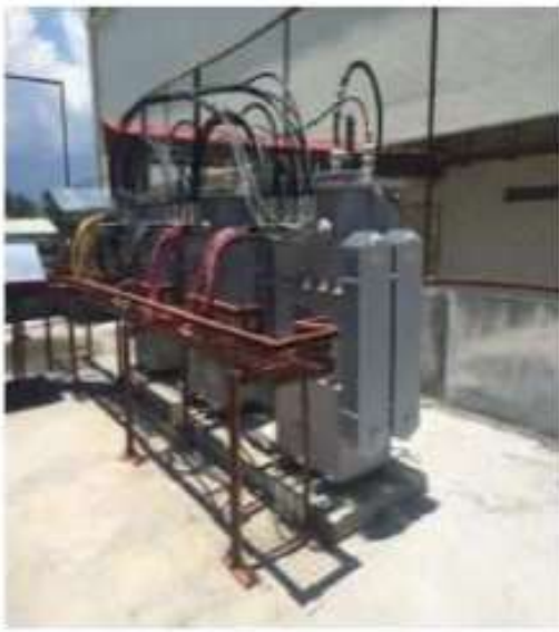
GAISANO TORIL – TRANSFORMER CONNECTION INSTALLATION
