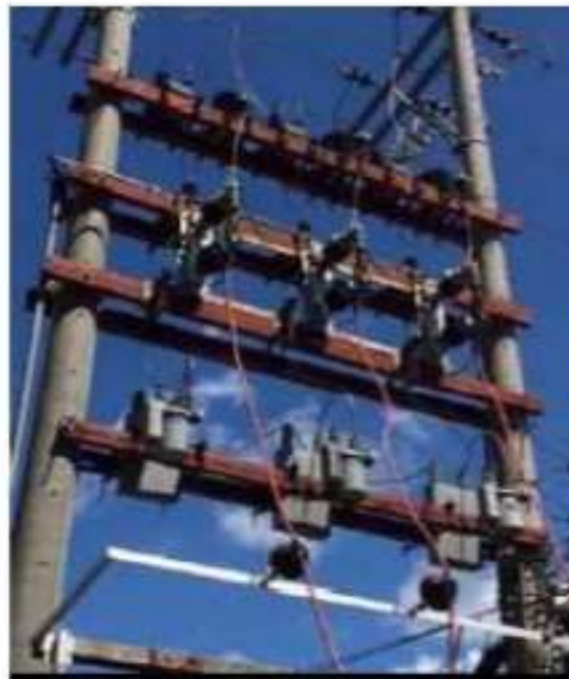
PRIMARY METERING INSTALLATION AT
