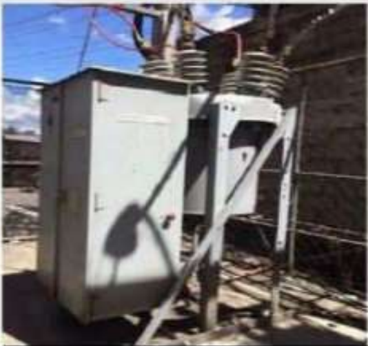
INSTALLATION OF 15kv, 1200AMPS OIL CIRCUIT BREAKER AT GAISANO MALL OF
